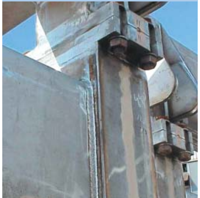
Dissimilar joint weld 3F, welded with BÖHLER CN 23/12 Mo PW-FD
